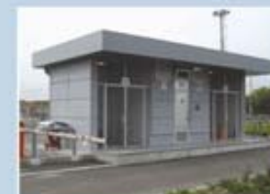
LPG filling station
